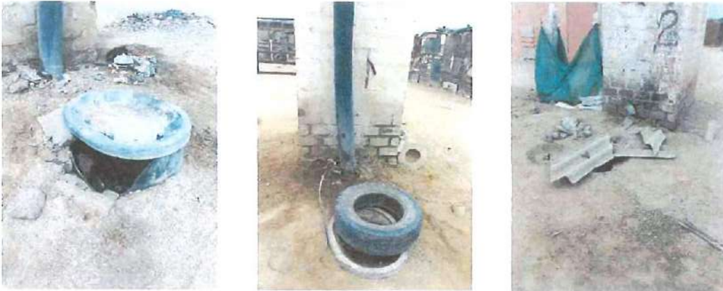
Figure 3. Damaged septic tanks
