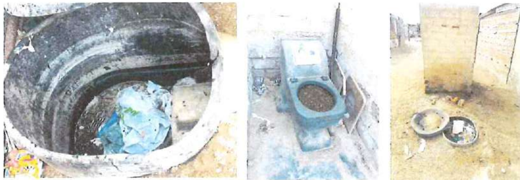
Figure 2. Full tanks that are not emptied and tanks with no lids
