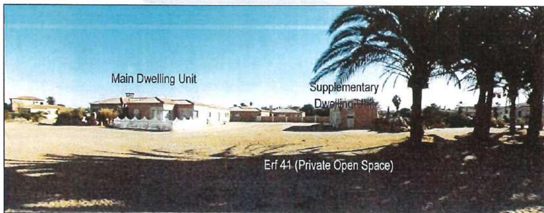
Figure 7: Photo of the open space between the main and supplementary dwelling unit as viewed from the east.
