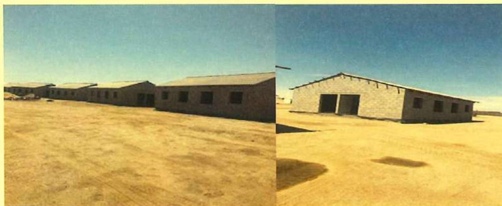
(Construction on Portion 48)
