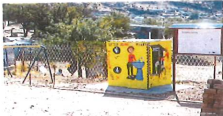
A demonstration toilet and sanitation centre in Oharyangwa informal settlement
