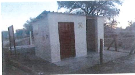
Finished sanitation centre in Katima Mulilo
