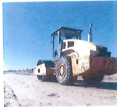
Road construction in Ohahave
