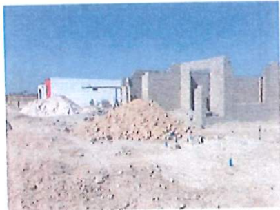
Houses being built in Ohahave
