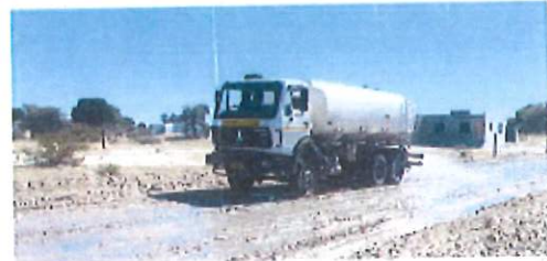
Road construction in Okahao
