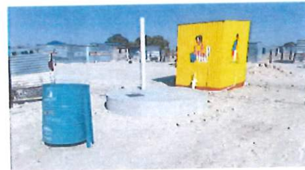
A sanitation centre under construction in Oshahoti
