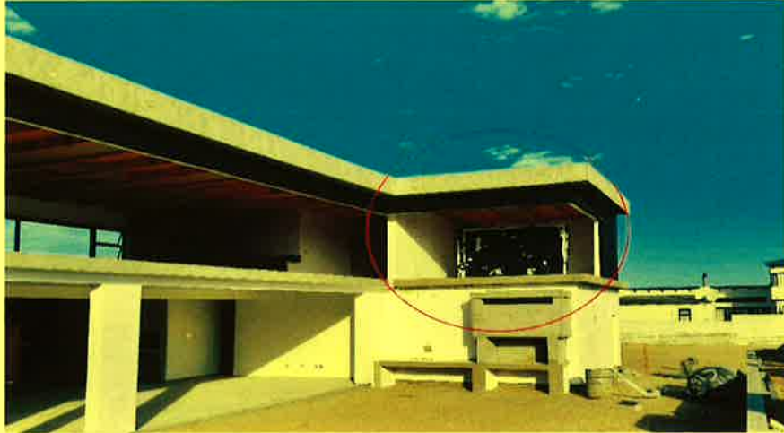
Figure 2: Structure built on the street at zero meters (0m)
