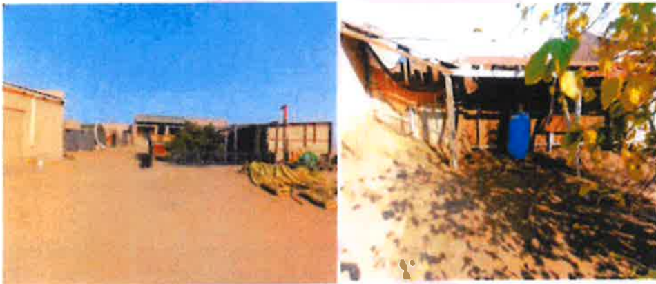
Figure 10 & 11 Photos showing Agricultural building on the left and a chicken shed on the right
