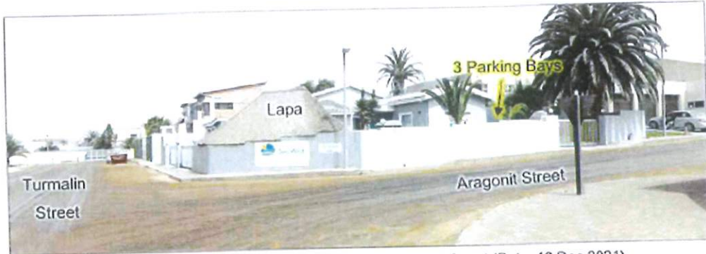
Figure 6: Photo of the site from the corner of Turmalin and Aragonit Street (Date: 16 Dec 2021).
