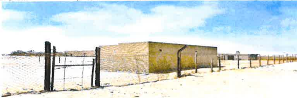
Figure 9 Current infrastructure and buildings on Portion 96 that were previously used for the oyster farm project
