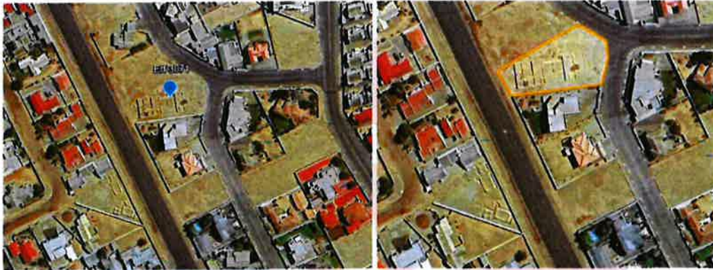
Figure 2 & 3: Aerial Photos of Erf 3071 Swakopmund Extension 9 and surrounding area.
