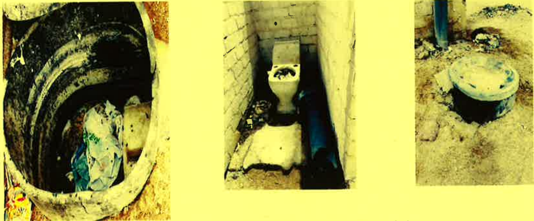
Figure 1: Full tanks that are not emptied and tanks with no lids.
